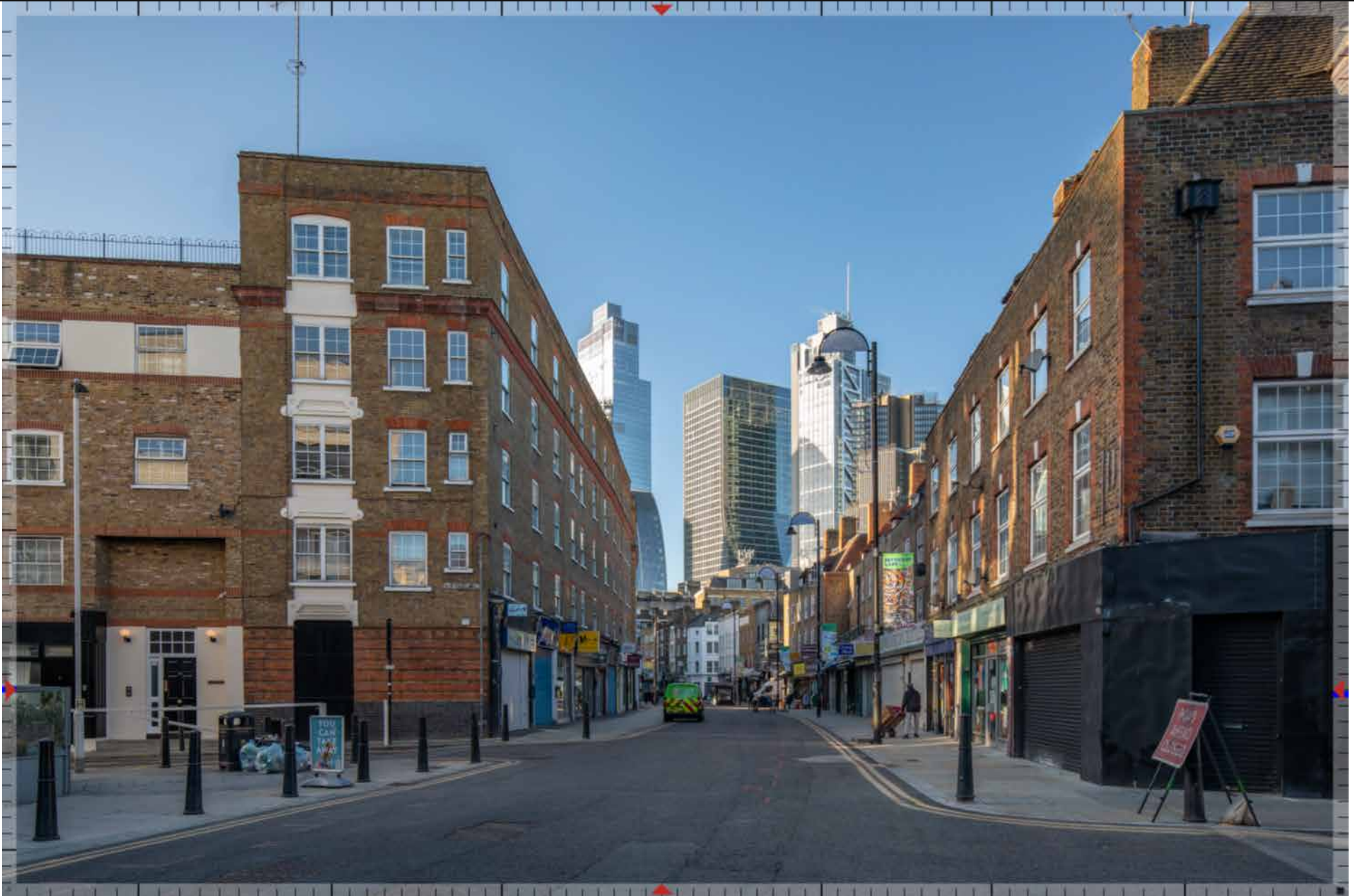
40 | Wentworth Street, corner with Toynbee Street
