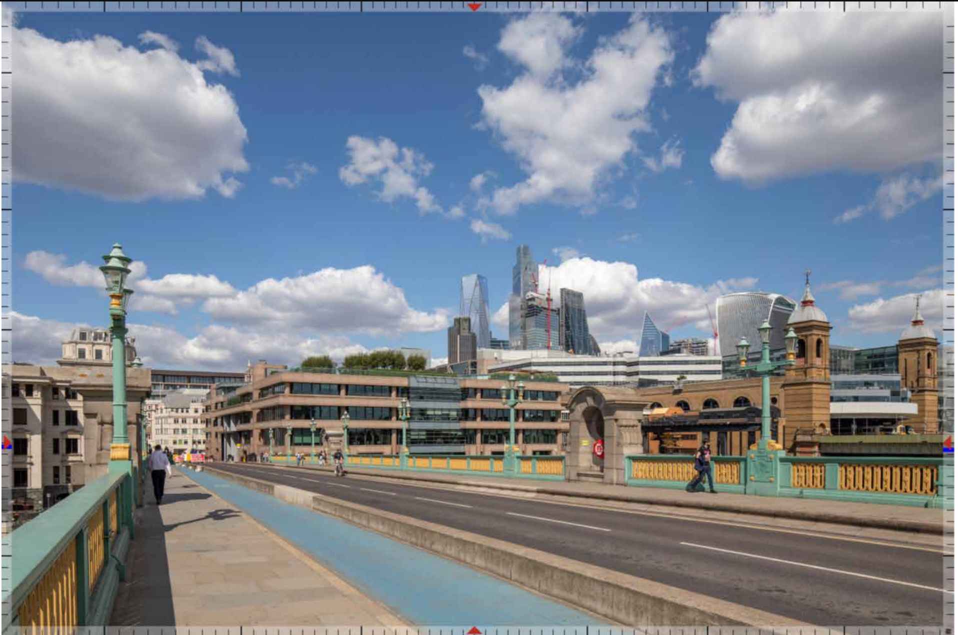
C04 | Southwark Bridge: LVMF 12A.1 position – centre of the bridge
